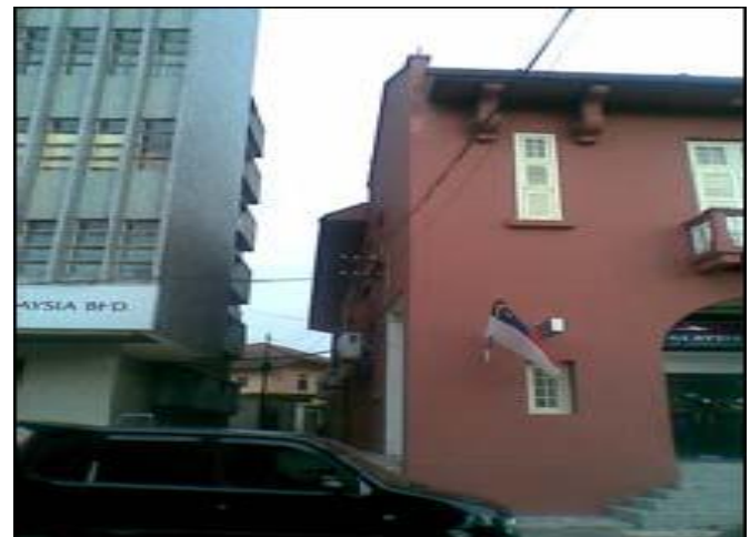
Figure 1 – A closely spaced building without setbacks
